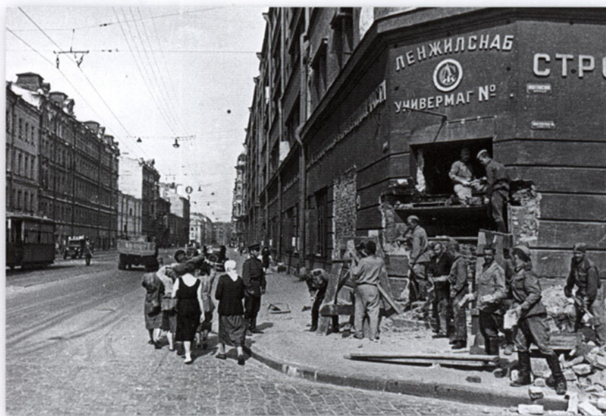
A department store on the Starinevski Prospect under conversion to a fortified gun position in September 1941. Leningrad's internal defences were strengthened with a series of anti-tank barriers, bunkers and hidden gun positions, which would have made a German assault into the city a very costly operation. (Fonds of the RGKFD, Krasnogorsk)
